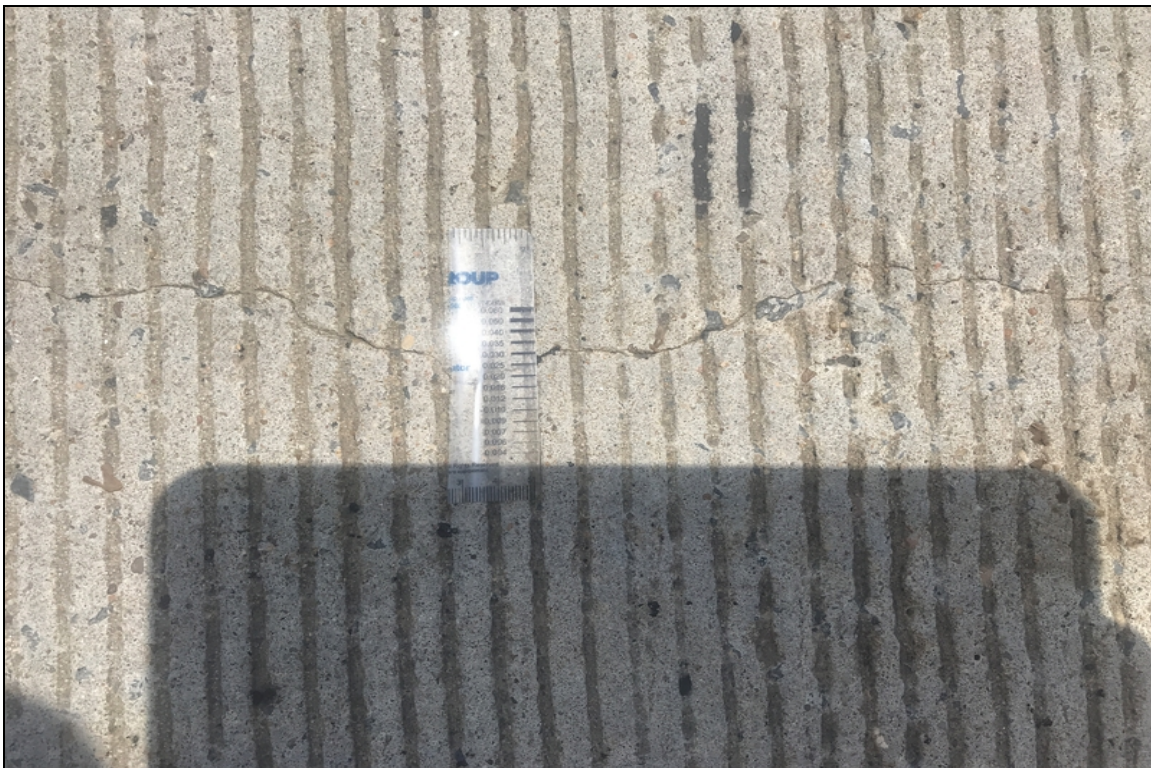
Deck cracks.
